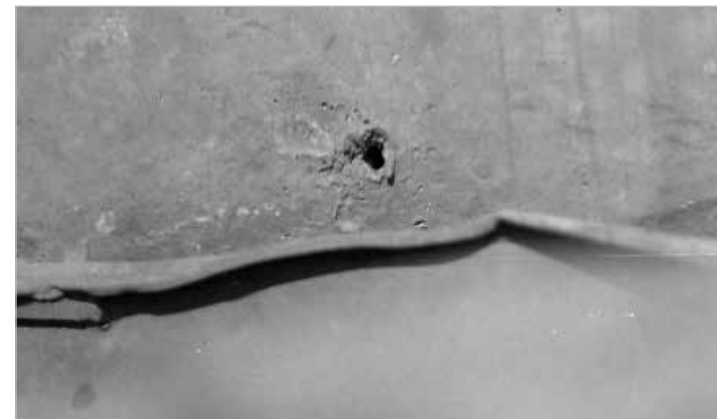
There is still an RPG hole in the side of the turret
